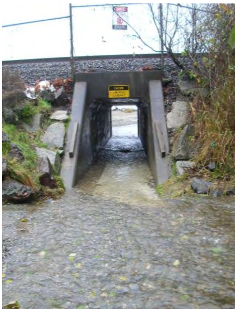
Figure 1: Meadowdale Box Culvert
